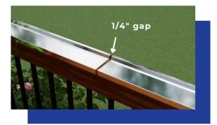
The minimum gap between rail pieces is 1/4" and the maximum gap is 1".
